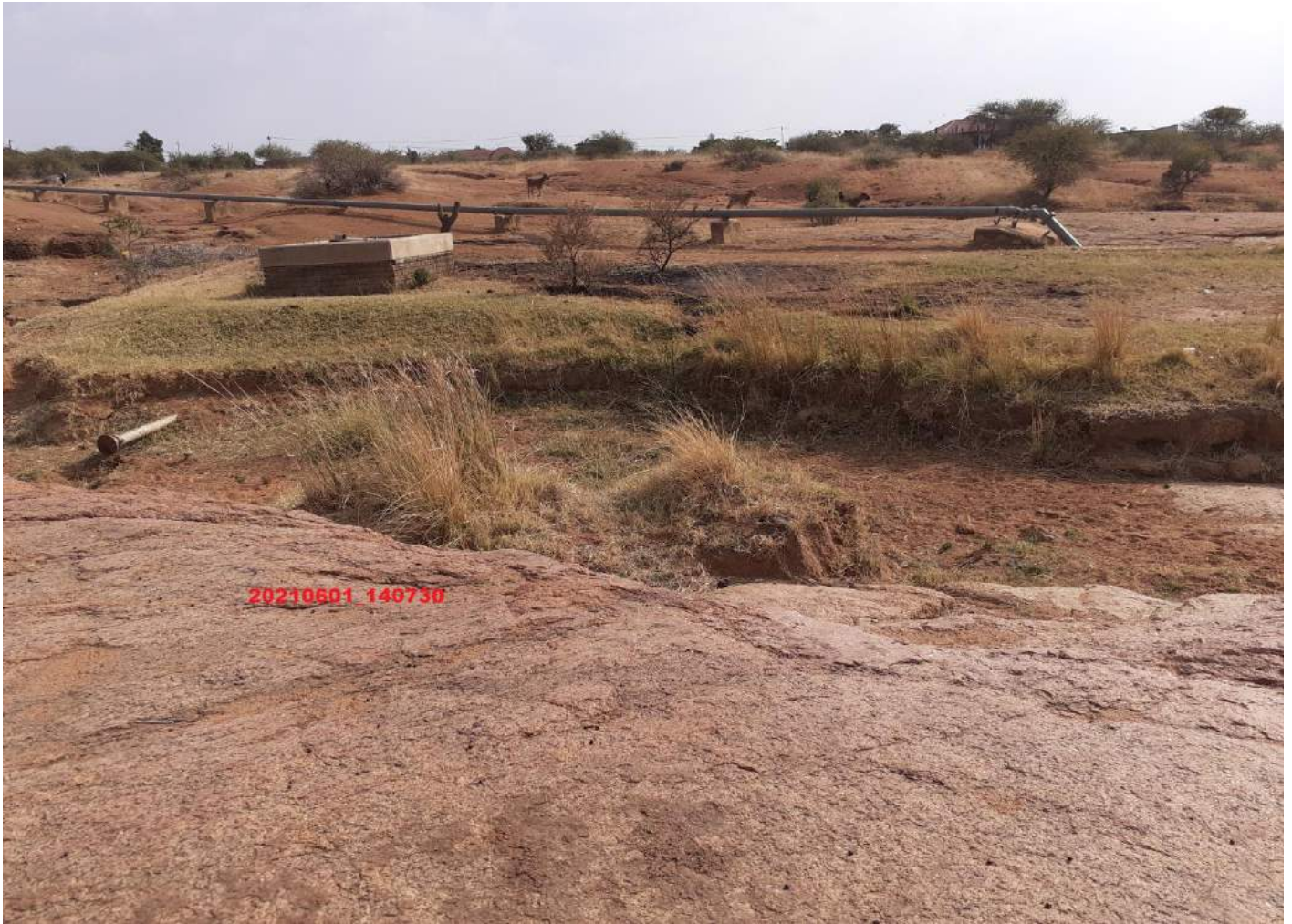
VIEW OF THE PUMP STATION UPSTREAM THE QUARRY
