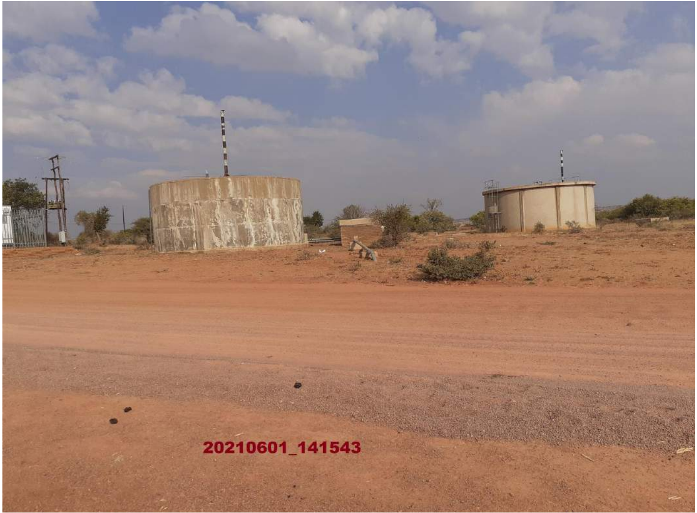
VIEW OF THE RESERVOIRS AND ESKOM SUB-STATION
